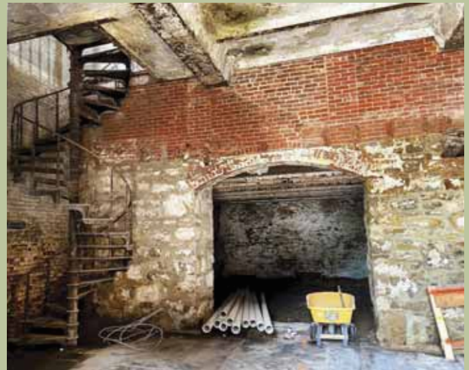
A look inside the arched front entry reveals a similar interior arch and at left, an iron circular staircase.
