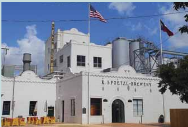
The Shiner brewery (top) as it appeared when first built in 1909. The Mission-styled structure above is reminiscent of the nearby Alamo and was built in 1947 as part of a major expansion effort. Today, the brewery uses it as a visitor’s center and taproom, with more contemporary buildings attached to it to handle modern machinery and increased brewing capacity.
