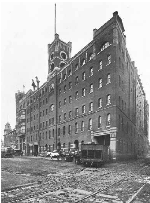
The Betz Brewing Company, c. 1905, Crown and Callowhill Streets, Northern Liberties, Philadelphia: the Crown Street front looking south from Willow Street.
