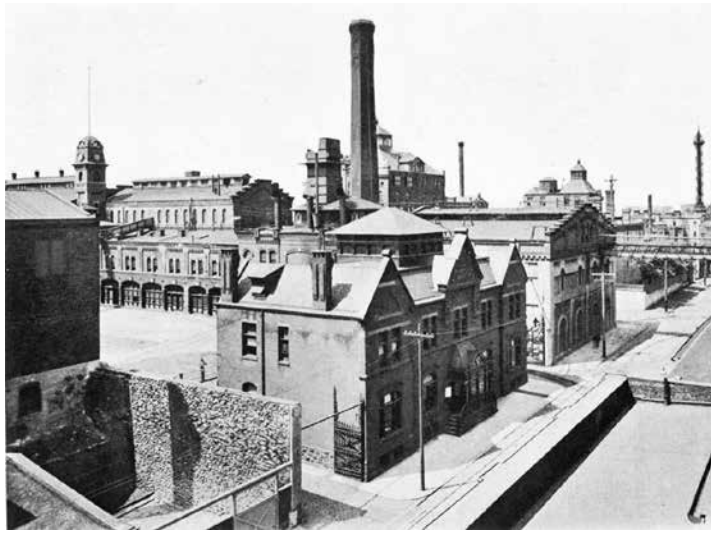
The Bergner and Engel Brewing Company, c. 1905, 31st and Master Streets, Brewerytown, Philadelphia, looking south from Master Street. (If the view was taken looking north the Poth Brewery would be visible in the background). This photo highlights similar decorative galvanized iron cornices, octagonal brick smokestack, and eclectic sampling from a variety of traditional styles.
